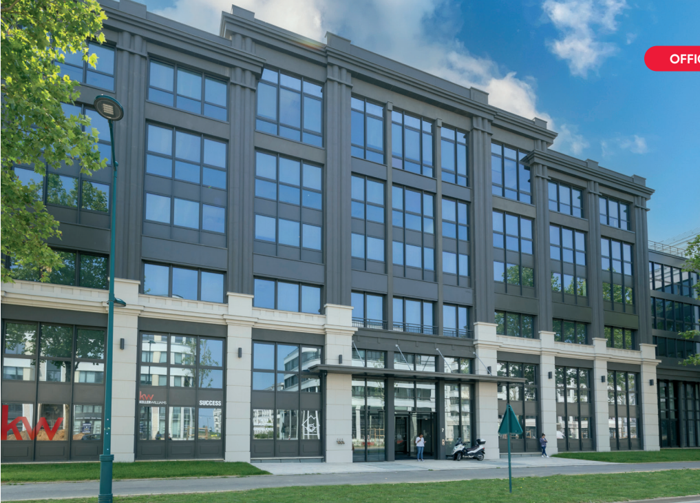
MayFair office building in Chessy (Legendre Immobilier)
