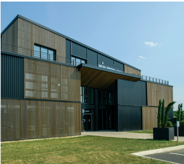
Digital Engineering School in Ferrières-en-Brie (Accelis)
