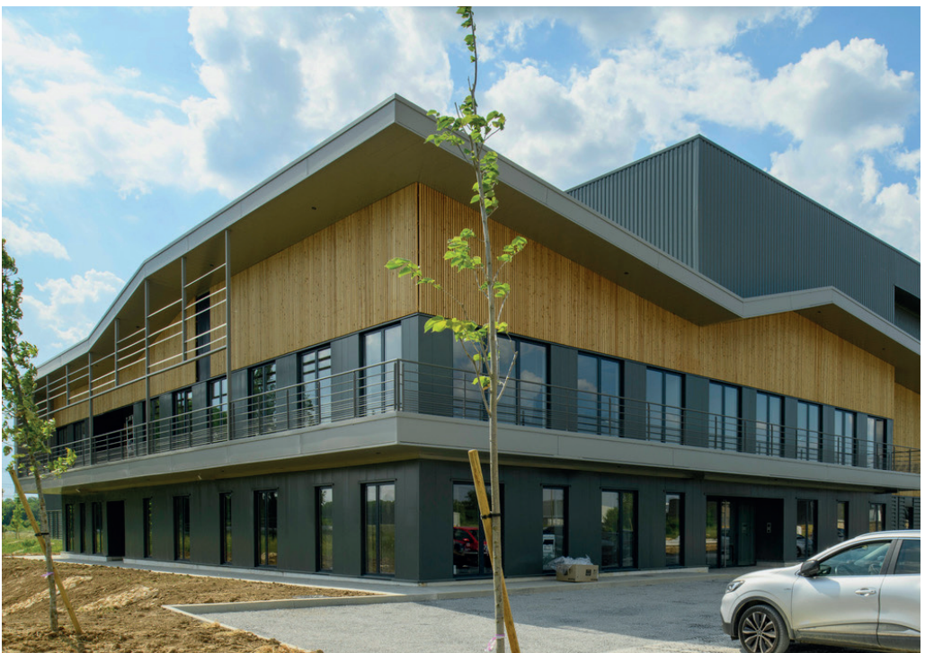
Guilbert Express building in Croissy-Beaubourg
